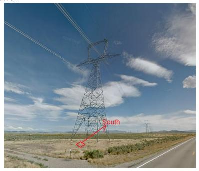
The OPUS result was not horrible. For the record: these are 500 kilovolt DC lines, not AC; so it could be worse. But in any case, you should avoid locations that are under transmission lines and have large steel towers directly to the South.
